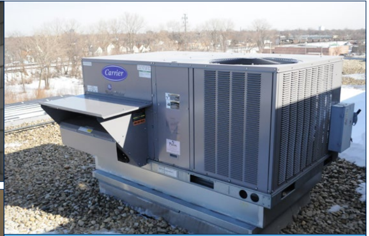
Figure 8: Fifteen high-efficiency gas-heat/electric-cooling units were installed.
