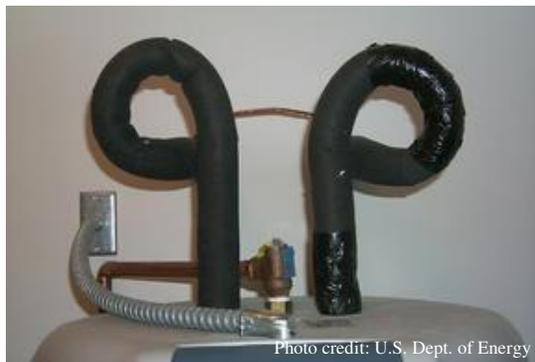
water heaters come with integral heat traps already installed so no additional plumbing will be required. For all other water heaters an external heat trap will need to be installed.
