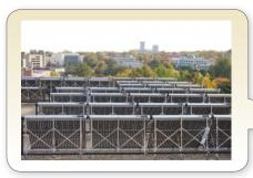
and the building will receive free solar thermal energy to keep hot water flowing in the building. The thermal panels, estimated to function for 30 years, trap at least half — and potentially all — the energy necessary to run hot water in the building, significantly reducing the amount of natural gas used. So far, residents have seen a 19% drop in their water heating bills.
